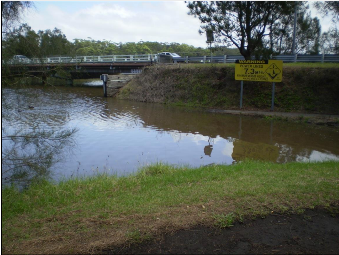
Figure 4: Flooding of the pedestrian underpass at the Crooked River Road Bridge, Gerroa in January 2012
