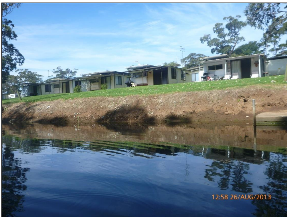
Figure 11(c): Areas of exposed bank in Blue Angle Creek
