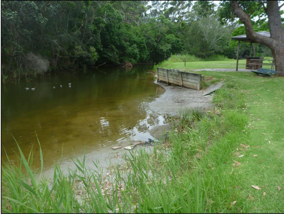
Figure 11(d): Erosion occurring in Blue Angle Creek
