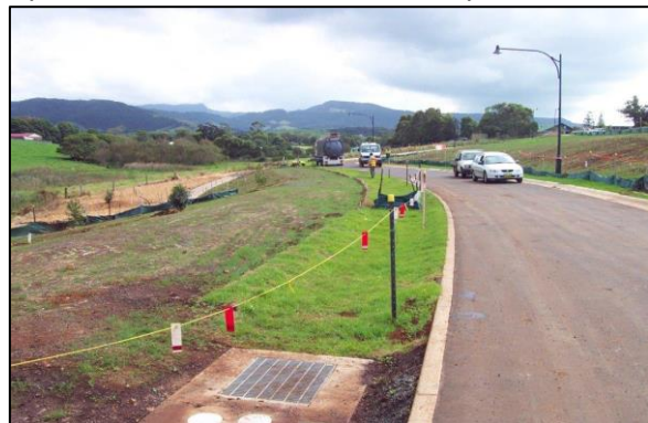
Union Creek riparian works in Elambra Estate
