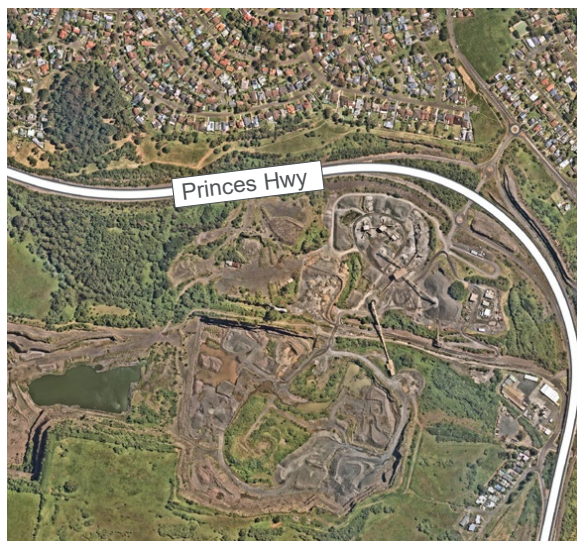
Figure 2 Above: Greenfield site in Bombo as identified in the LSPS Below: Aerial map of the Bombo Quarry
