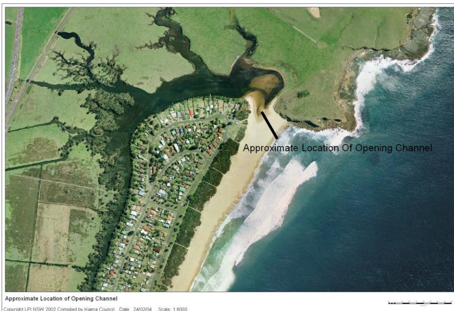
Figure 5: Location of Werri Lagoon entrance channel (solid line indicates area for location of excavated channel).
