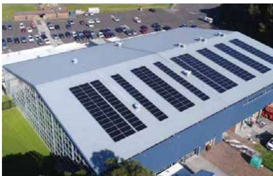
Figure 2: Solar panels on the Kiama Leisure Centre, Source: Kiama Municipal Council
