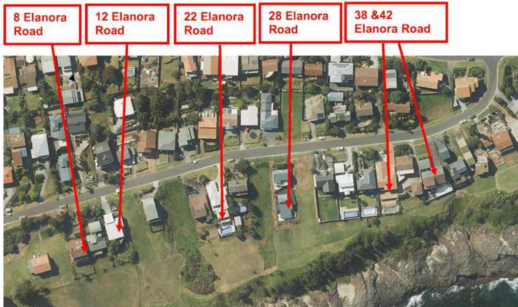
Aerial view of affect dwelling on Elanora Road
