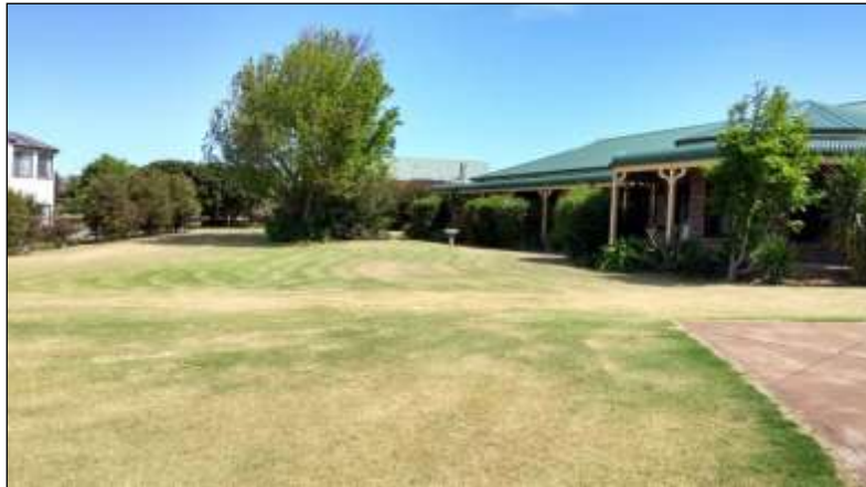
Figure 5 – Site Photograph – Existing Single Storey Dwelling
