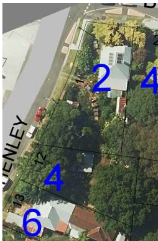
Figure 3 – Site Photograph (↑N, 2016 View)
