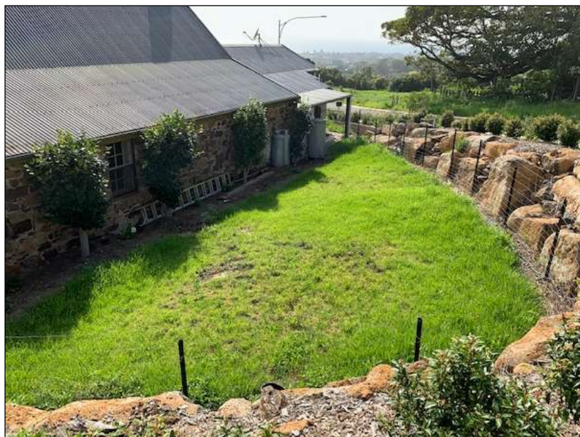
Figure 5 – Photo Taken from location of Cross Section AA
