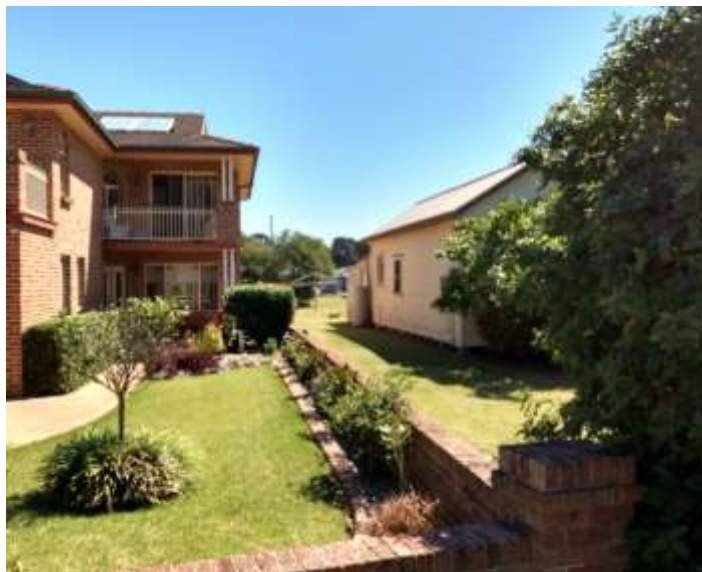
Figure 4 – Site Photograph (South-west View) – Propose Access Corridor Location
