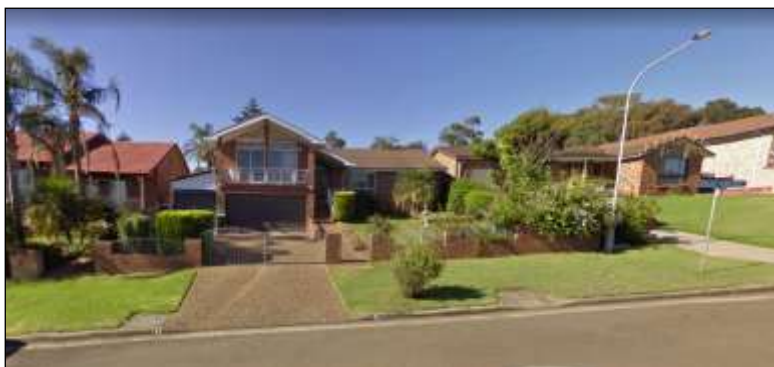
Figure 2 – Site Photograph (South View) – Existing Dwelling, Carport and Driveway
