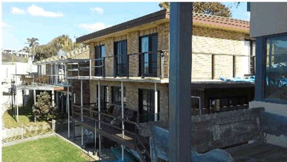
(view from upper level deck)
