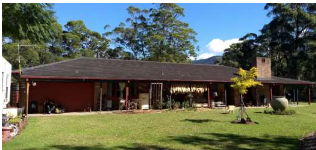
Figure 2 – Site Photograph (West View)
