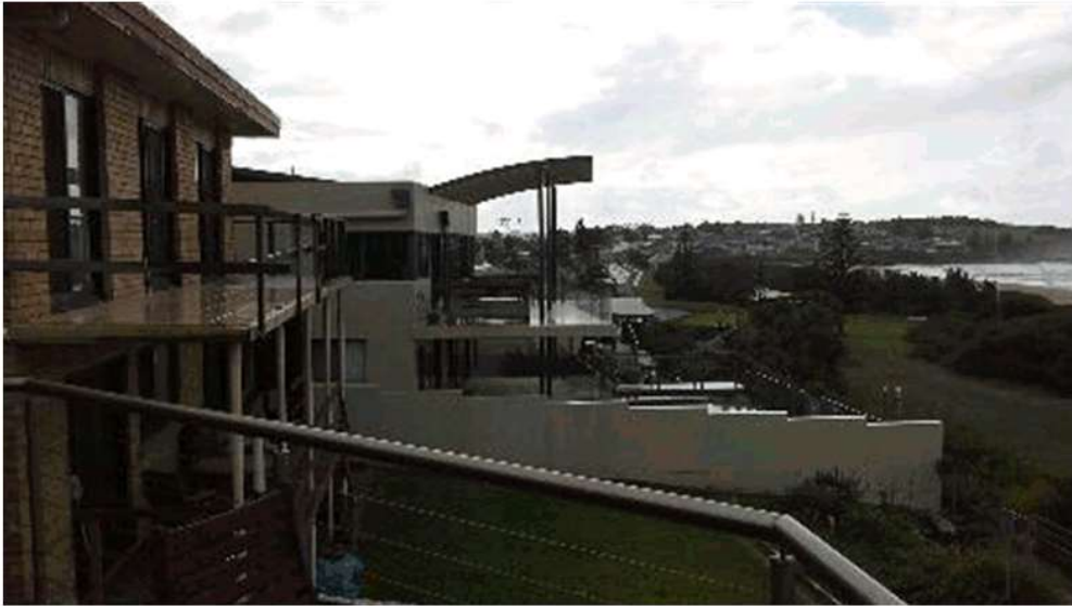
(view from upper level deck)
