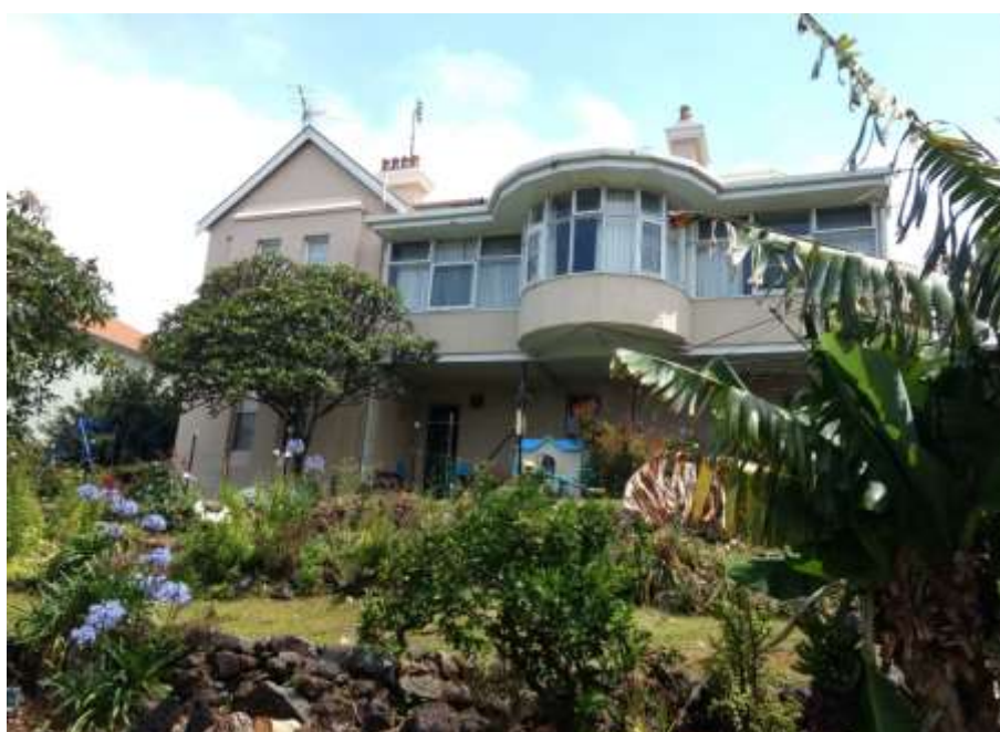
Figure 5 – Site Photograph – Rear of Heritage Item (South View)
