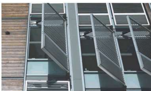
Building users should have the opportunity to open windows and operate privacy screens and sun shading devices from within buildings
