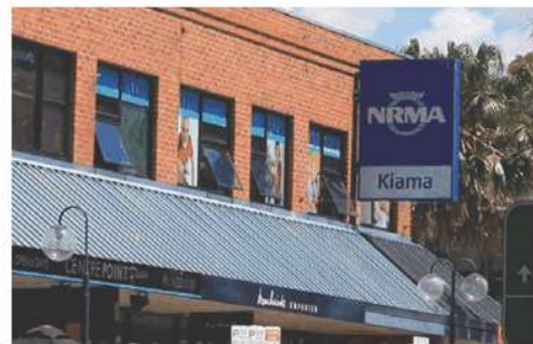
Intrusive signage such as the above example in Terralong St is recommended to be prohibited under the revised DCP
