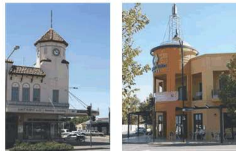
Example of corner elements - historic (left photo, Goulburn NSW) and contemporary (right photo, Mawson Lakes SA)
