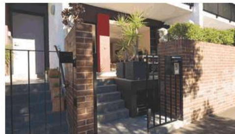
Example of an elevated residential dwelling on the ground floor that is directly accessed off the footpath
